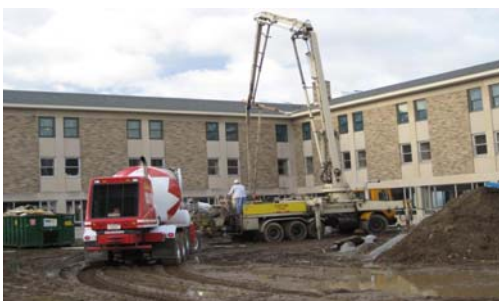
Just before the snow the parking lot was paved.
