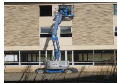
New windows are being placed throughout the building.
