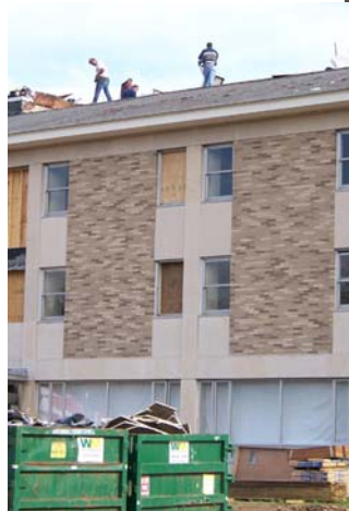
Men working on the roof replacing the slate.
