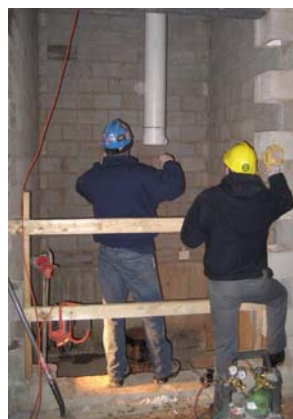
The cylinder for the elevator is put in place by the crane. Workers in the elevator shaft guide it into place.
